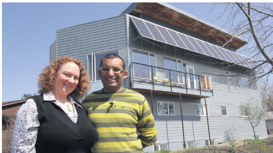
Shafraaz and Serena Kaba with their three-storey, near-net-zero home that is super energy efficient and tailor-made for the climate of Edmonton, Canada's most northerly big city. DAVID DODGE, GREEN ENERGY FUTURES
